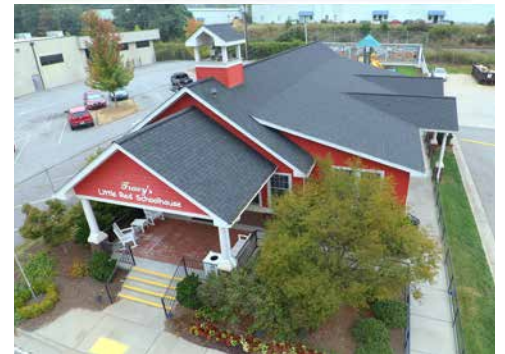
Tracy's Little Red Schoolhouse then and now – thank you to Shelco, LLC.
